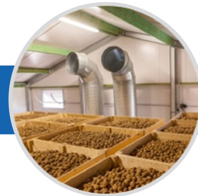
Ventilation of warehouses, sheds, storage facilities
