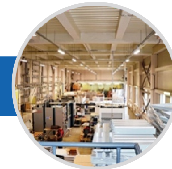
Ventilation of production rooms
